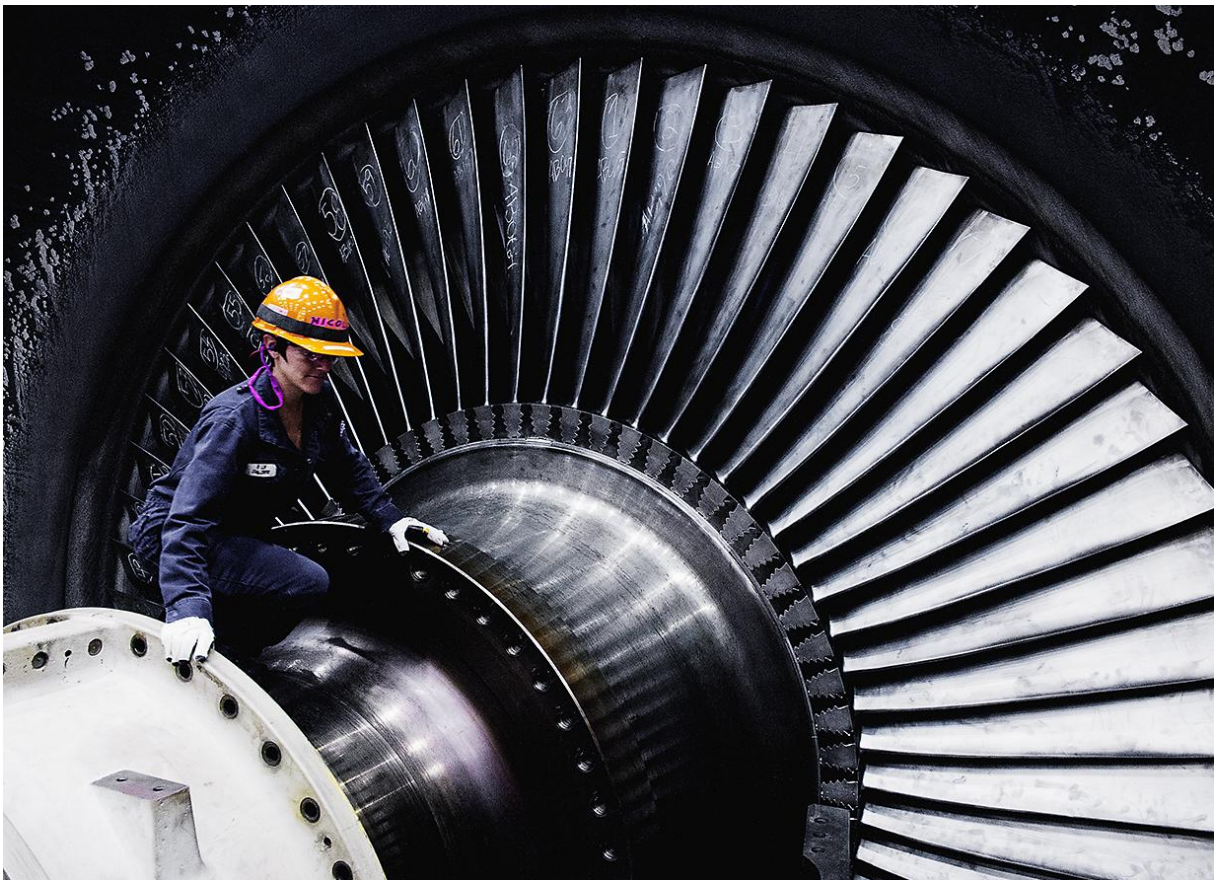
Photo 4 - Inspection of Turbine Generator Blades
